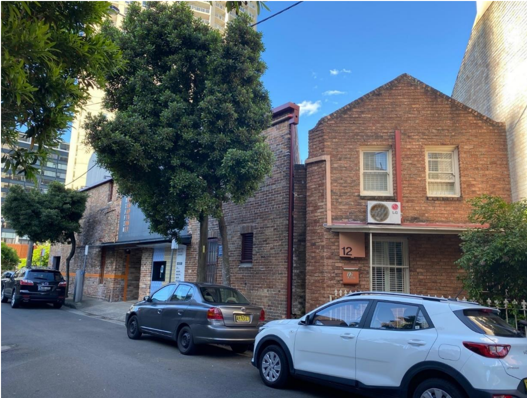
Figure 5. 10 and 12 Nimrod Street viewed from the south-west
